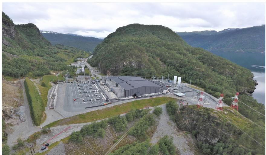
The North Sea Link (NSL) interconnector between Norway and UK: 1,400 MW, ±525 kV, 730 km
