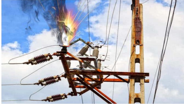
Typical faults (shortcircuits)
